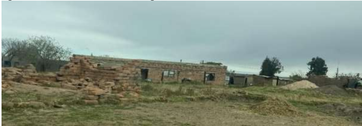
Figure 5: Blaauwbosch Houses Built Using the Bricks Produced from the Mine
