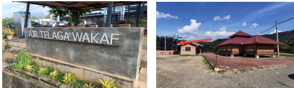
Figure 4: The construction of Waqf Water Wells in several locations in Kedah and Pahang
