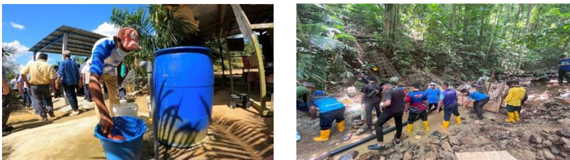
Figure 5: Construction Works of Waqf Water by Yayasan Waqaf Malaysia
